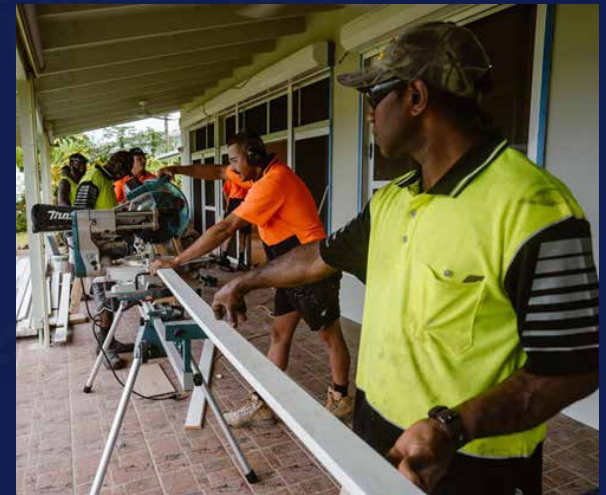
Australian High Commission Residence, Port Vila Vanuatu
