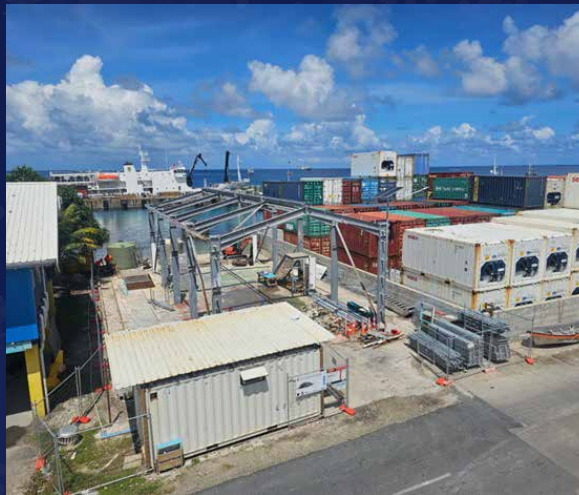
Tuvalu Police Maritime Wharf & Workshop Upgrade
